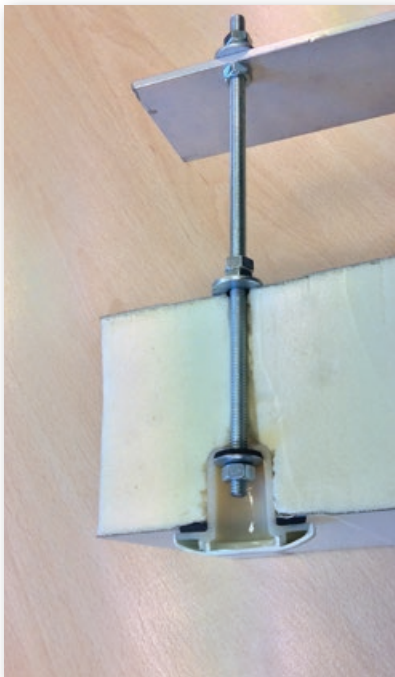
Suspension of the ceiling panel on a threaded rod directly to the structure
